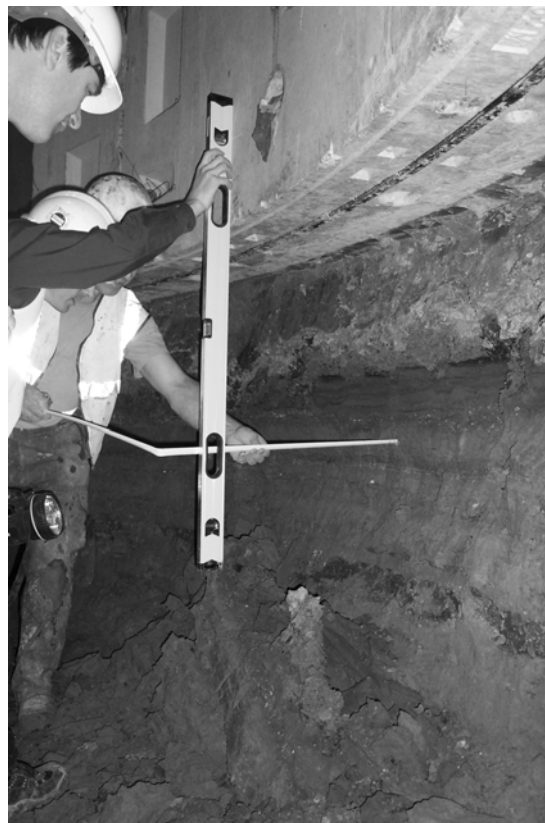
Figure 14 Silty sand slumping from the excavated face during ring build in water bearing layer in Upper Lambeth Group
