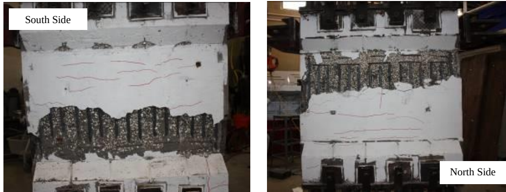
c) Failure of OPR
