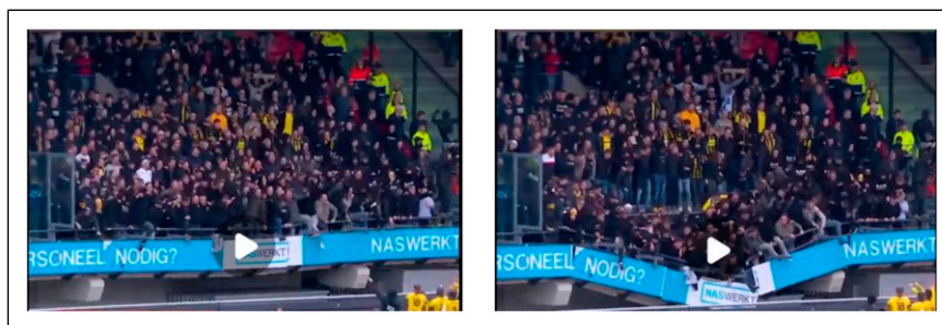
Figure 1. A grandstand collapsed due to jumping spectators. ( https://www.bilibili.com/video/BVIRrK6zMESi/?vd_source=156cd4cd2e8750e749736923f801e9f2 )
