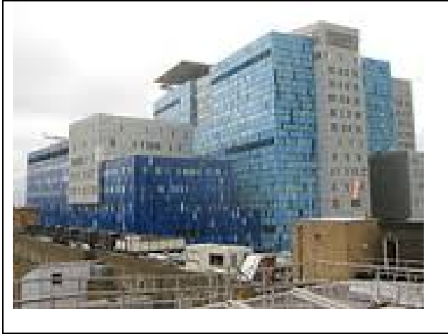
Figure 19- The New Royal London Hospital PFI building
