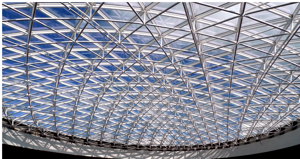
Figure 3: Arrangement of structural members and connections following a regular pattern in a spatial structure. Image reproduced with permission from Geometrica Inc.
