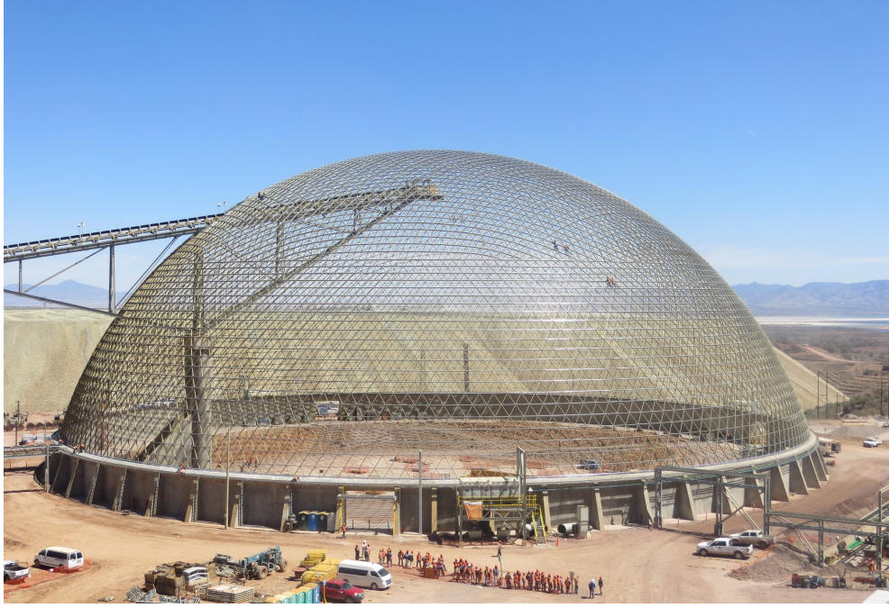
Figure 1: A single-layer lattice dome covering large span. The image reproduced with permission from Geometrica Inc.
