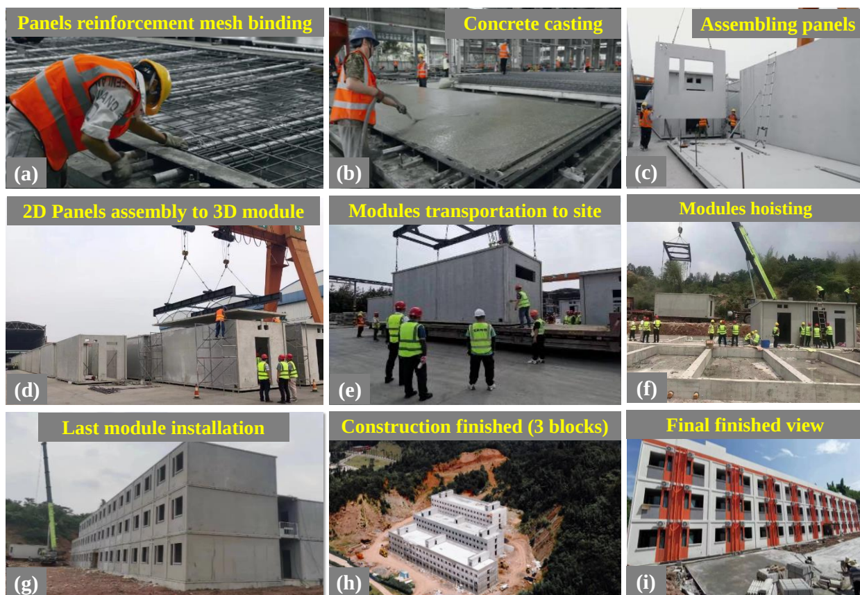
Fig. 1 Stepwise construction process of prototype PVMS with proposed IMCs
