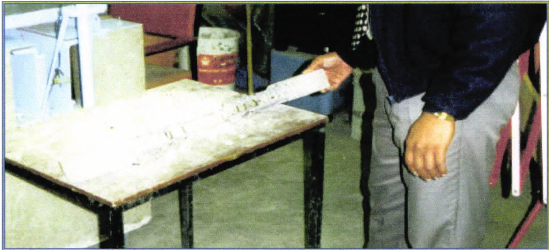
Figure 8.1.2d Typical explosive failures of reinforced concrete beams.
