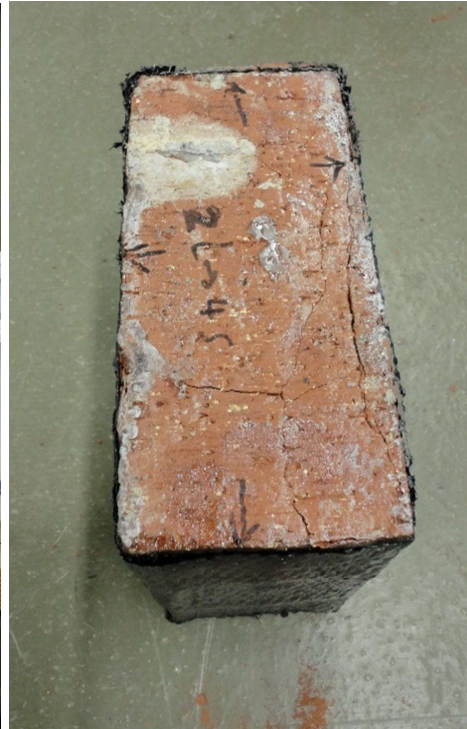
Figure 3.28: Strengthening with two-layer of CFRP wrapping on four sides
