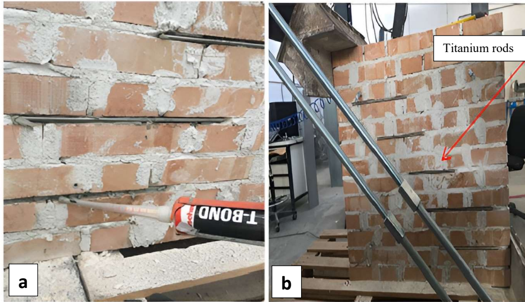
Figures 5.3a and 5.3b: A repaired wall panel using titanium rods for crack stitching, Corradi et al (2020).
