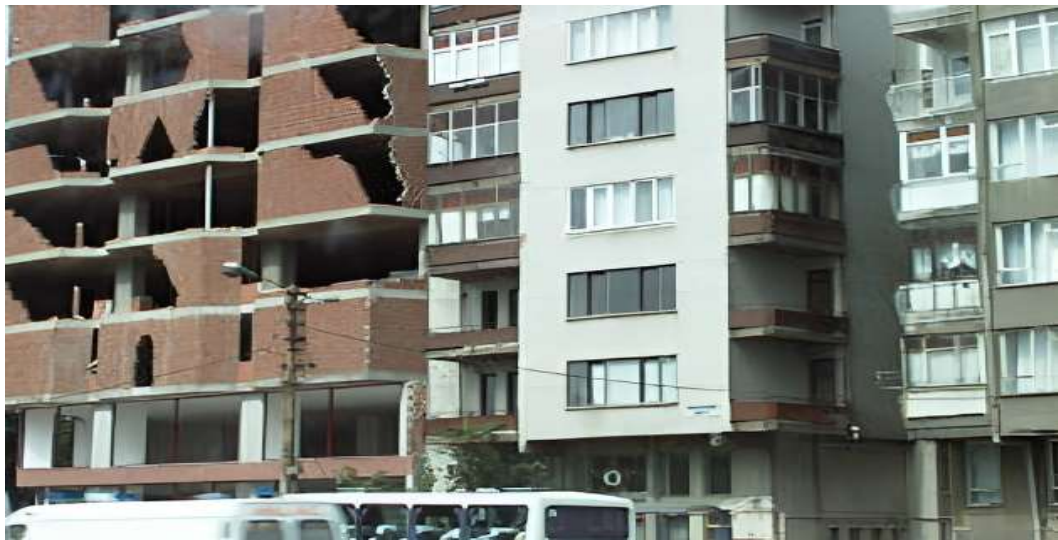
Figure 2.1. The collapse of URM Walls, Turkey, 1999. (Tumialan & Nanni, 2001).
