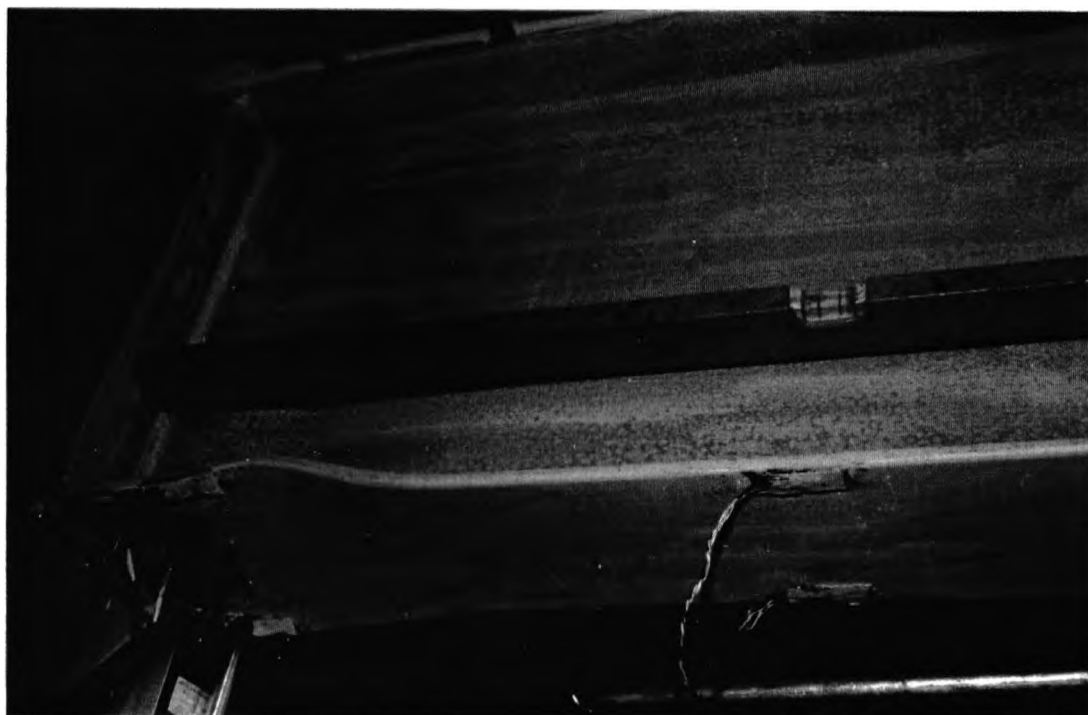
Figure 4.31 Sub-Assembly Ultimate Load Test 2 - Local Web and Flange Buckling of Beam B1
