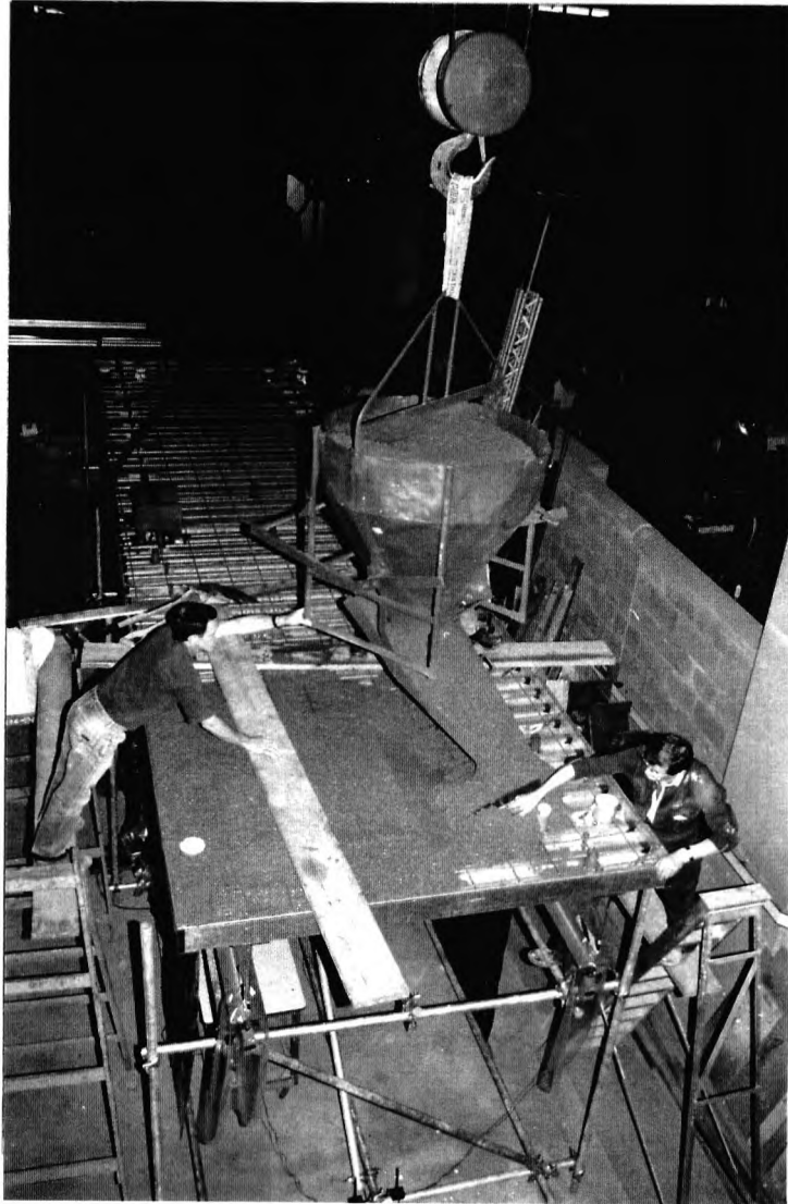
Figure 4.5 Sub-Assembly Test - Pouring the Concrete Slab
