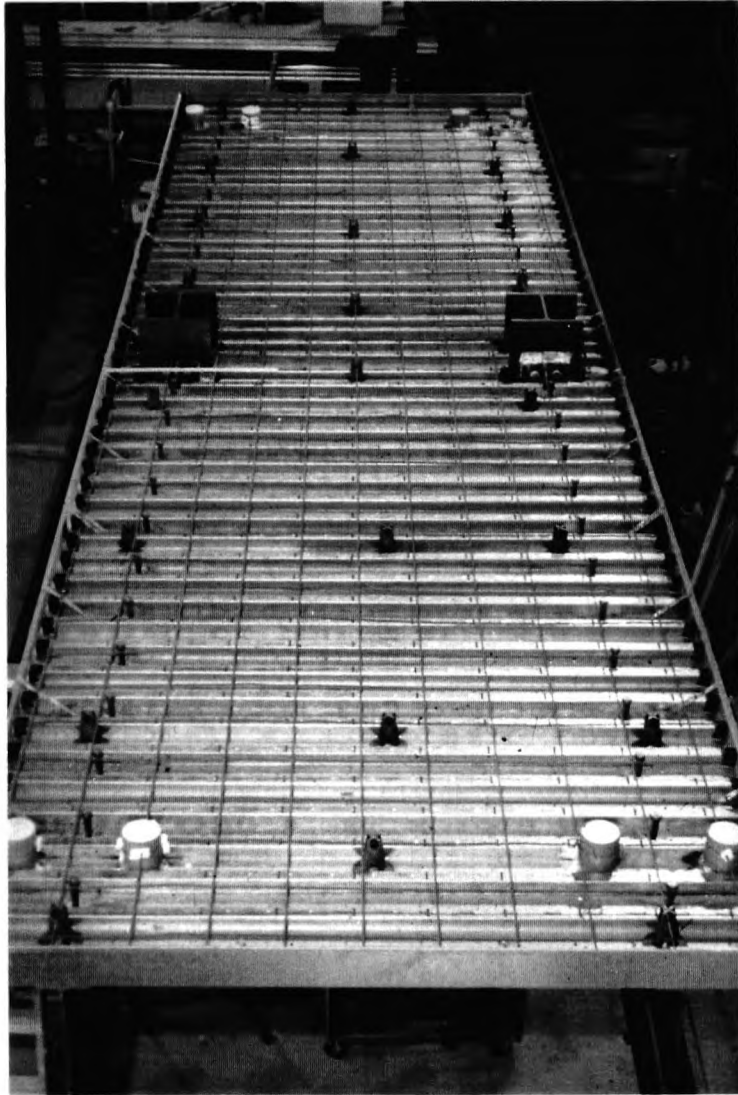
Figure 4.4 Sub-Assembly Test - Prior to Pouring the Concrete Slab
