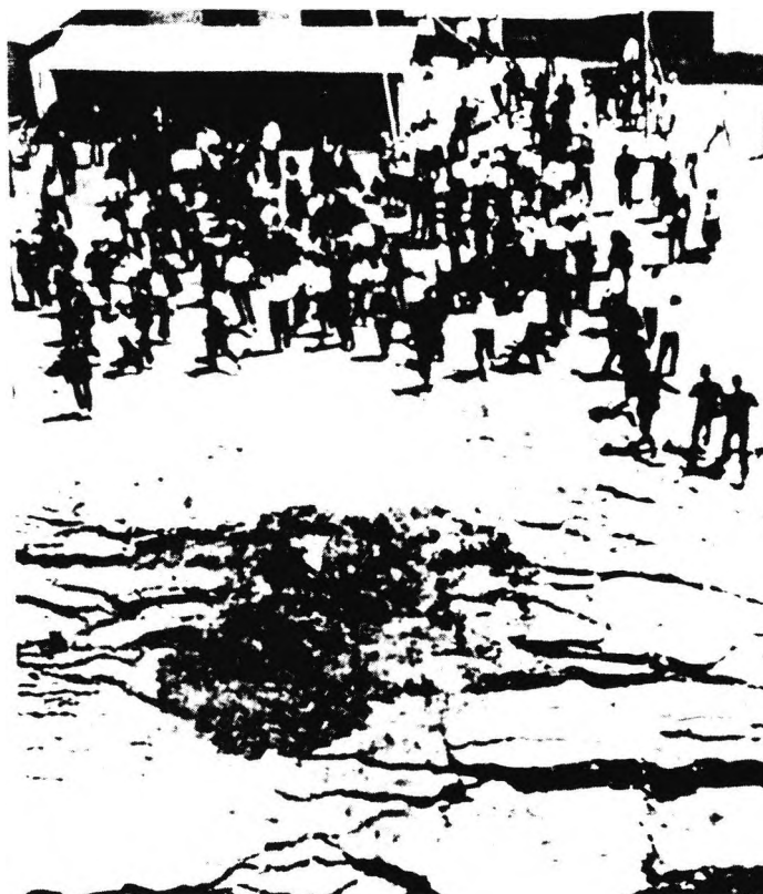
Figure 3.13 Ground cracking and initial flow of water at ground level, Niigata 1964 (after Seed, 1970)
