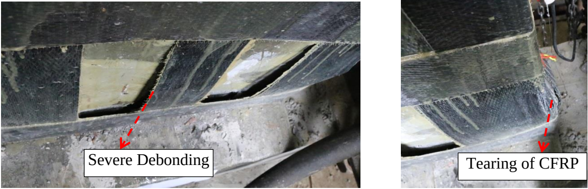
(a) (b) Fig. 13 Failure mode of repaired specimen RW4: (a) front view, (b) side view
