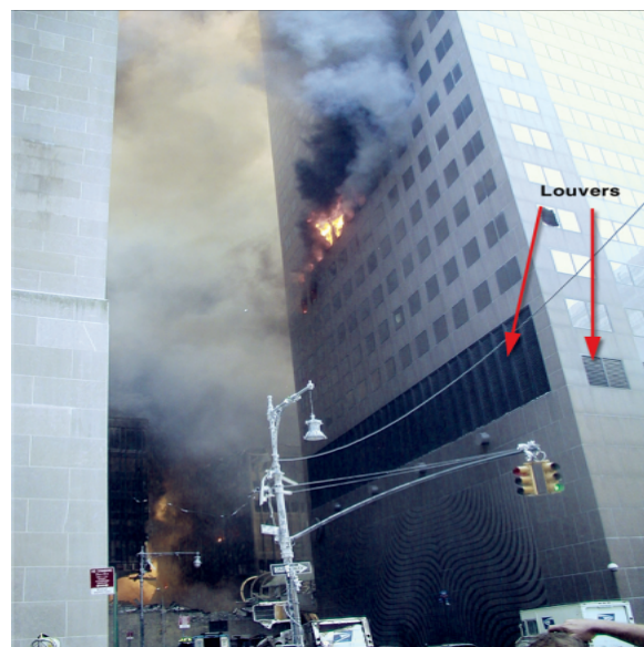
(b) Fires on the 11th and 12th floors of the east face of WTC 7
