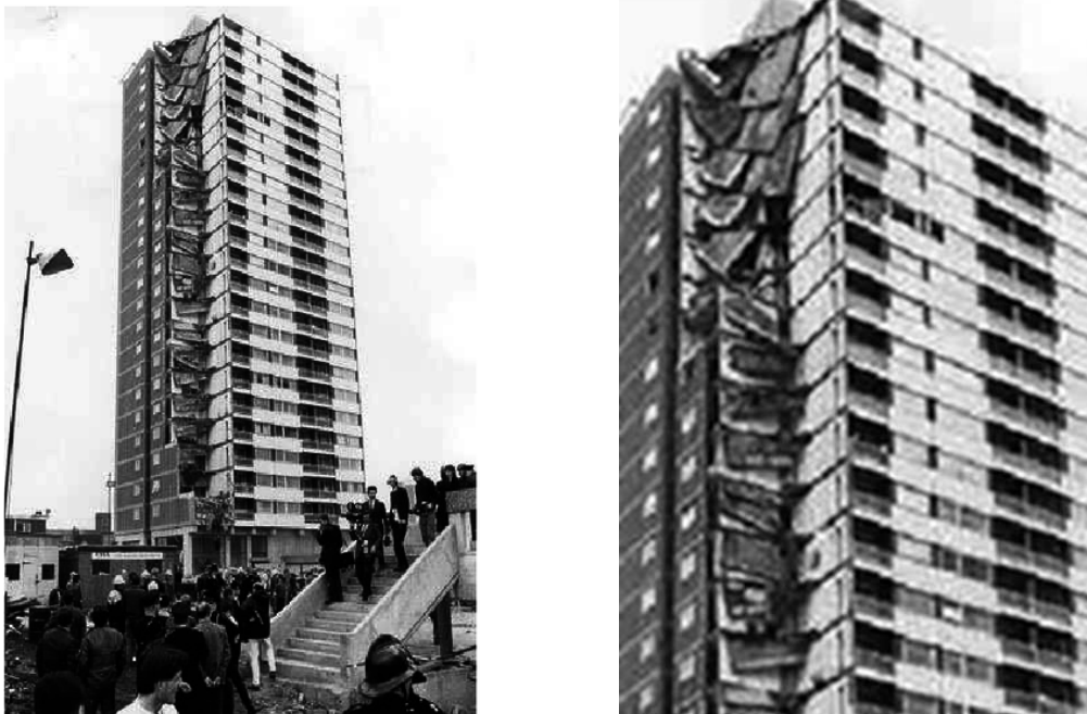
Fig. 2.1 Disproportionate collapse of Ronan Point (Pearson and Delatte, 2005)
