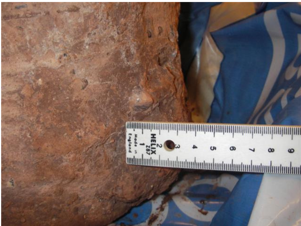
Figure 4.15 Aggregates from concrete of the pile coming out from the surface of the pile shaft. Pile MR1, 0-495mm below ground level.
