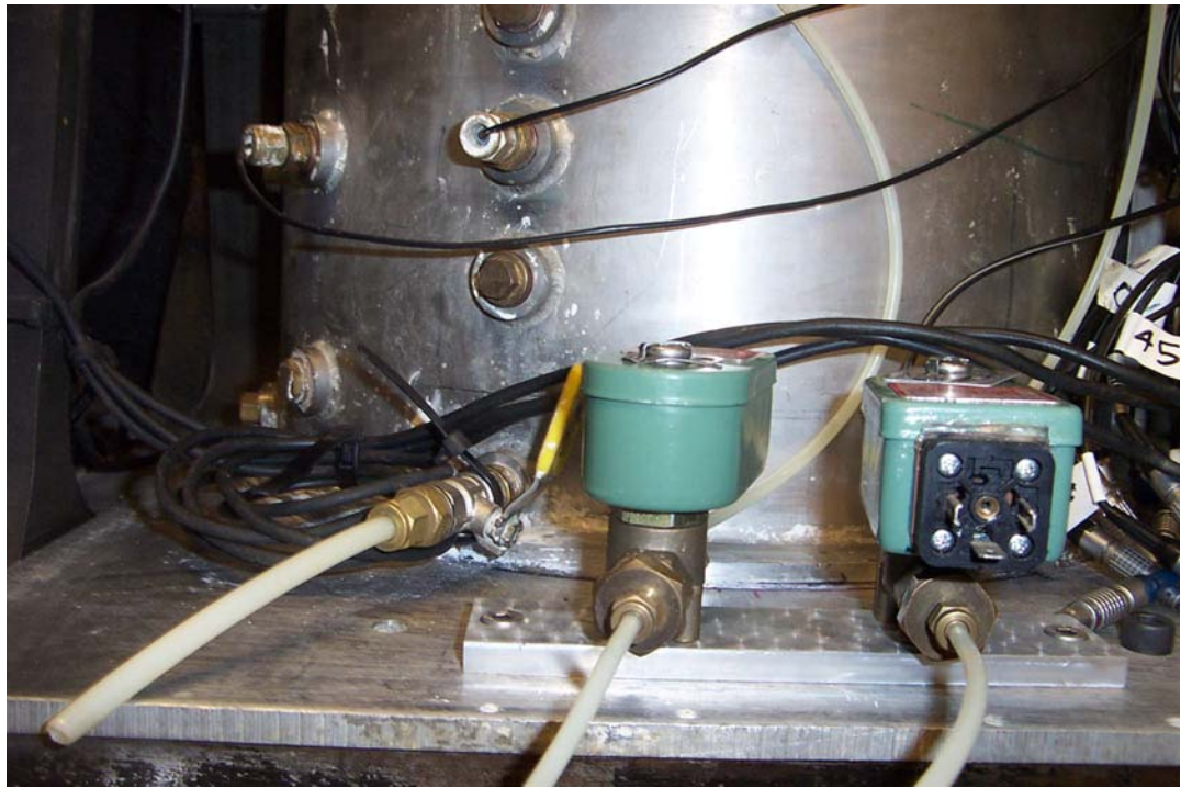
Figure 3.31 Solenoid valves used to drain the water from the loading reservoirs during foundation unloading.
