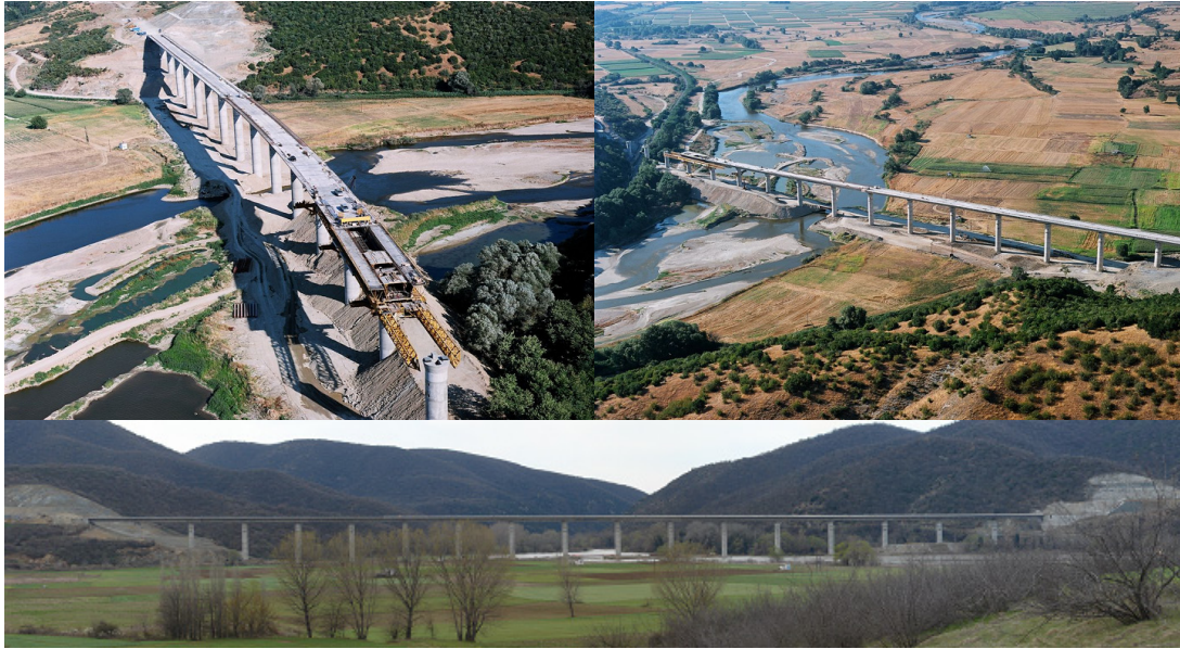
Figure 2: Various aspects of the T12 viaduct
