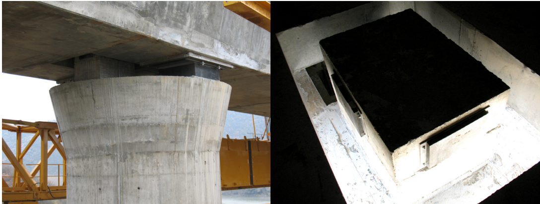
Figure 6: Pier Head and Stopper Details
