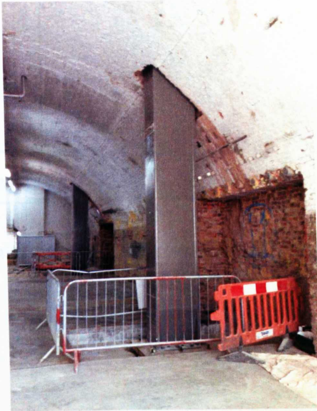
Figure 3.11 Structural column installed
