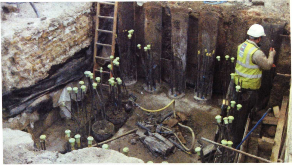
Figure 3.06 Cutting down pile heads to formation level
