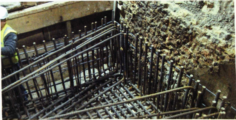
Figure 3.07 Installation of pile cap reinforcement
