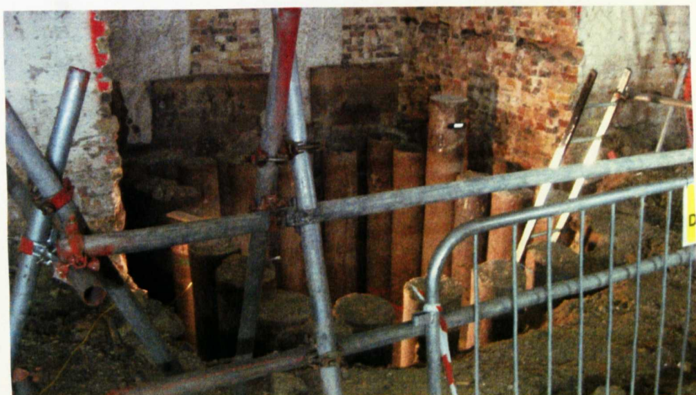
Figure 3.05 Excavation to pile cap formation level
